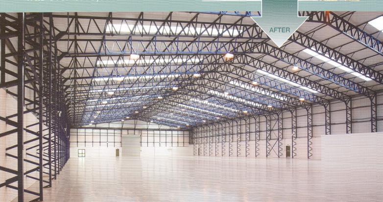
The refurbishment included the complete replacement of the elevations and roof cladding with new insulated profile sheet metal cladding; the removal of all internal structures which have been replaced by a new office and WC block totalling approximately 1,500 sq ft, new loading doors and a refurbished warehouse floor.
